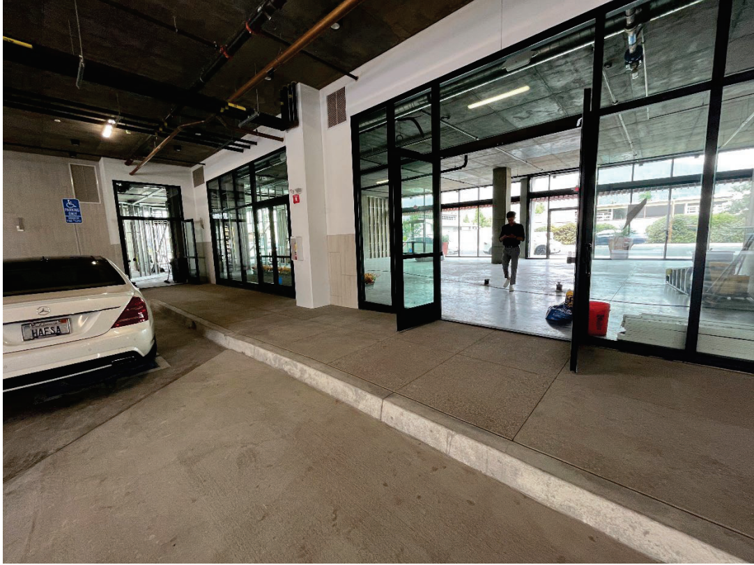
Entrance to the rear of the units from the parking lot
