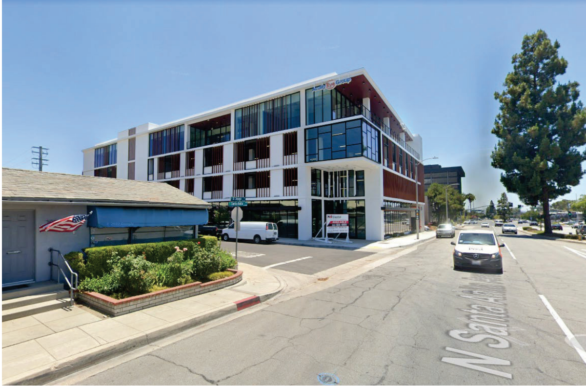
Looking south on N. Santa Anita Ave toward 288 N. Santa Anita Ave and the two units facing St. Joseph Street.
